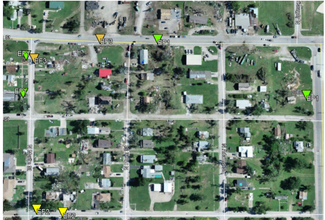
Eureka, KS Tornado June 26, 2018
